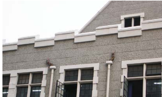
Fig.13 Parapet and Downspout
